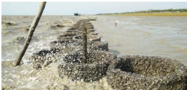
Figure 4b: Artificially Grown Oyster Reefs on Submerged Concrete (Source: Future Planet, 2021 [26])
