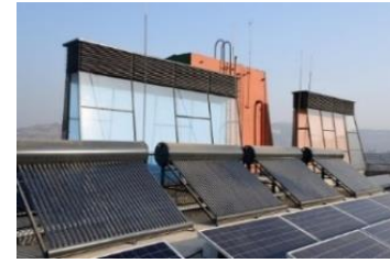
Figure 9: Photovoltaic Solar Panels and Solar Water Heater
