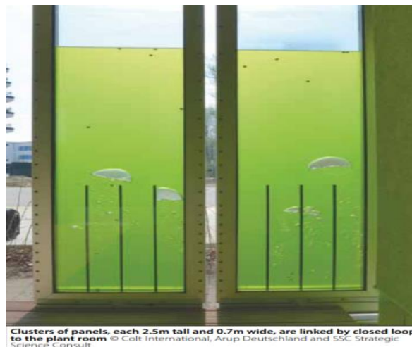
Figure 2: Cluster of Panels with Algae Solution within It
