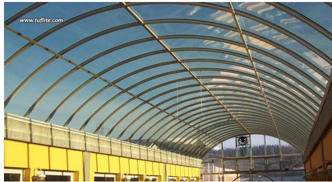
Figure 10: Aluminium Frame Combined with Polycarbonate Roofing Sheet Used for Roofing [xv]
