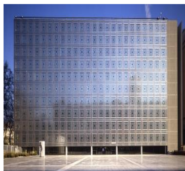
Figure 3: Moucharabiehs Screen having Mechanism
